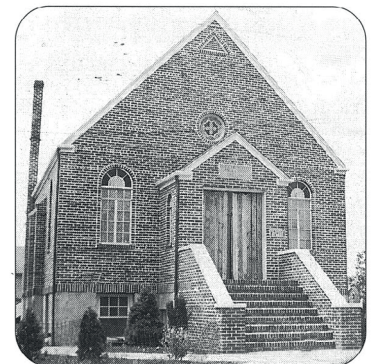
Hopelawn Church Building on Florida Grove Road
